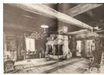
The oldest of these Finnish log houses were called "smoke houses" since their huge fireplaces did not have chimneys but instead allowed the smoke to drift upwards and out a "smoke hole" in the roof. It was an opening covered with a flap which was let down when the fireplace was heated and then closed by lifting it up
